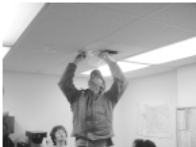
Joseph Mead seals a ceiling vent.
