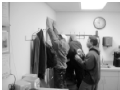
David Peres and Carlos Flores seal the door at Central Dock.
