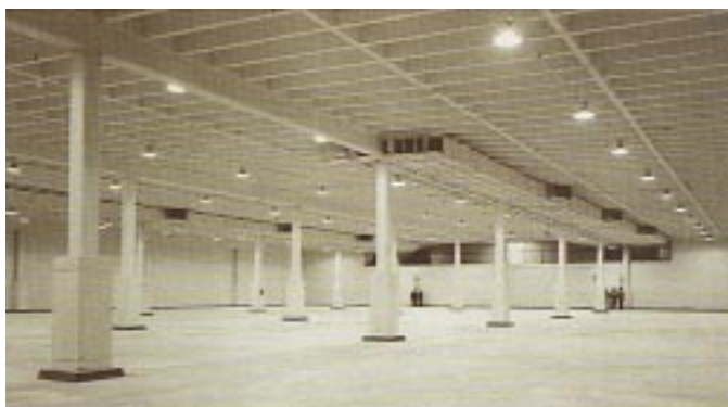
Warehouse 3 upon completion in 1954.
